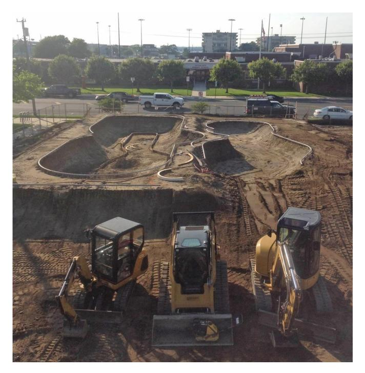
Task 3.4 Earthwork & Drainage – With the construction site established, Mark will lead the team as they clear the site, install the drainage system and contour the terrain.
