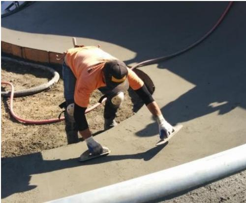
Task 3.6 Place **Shotcrete & Concrete** for Skate Elements/Terrain -Mark Bradford, an ACIcertified shotcrete nozzleman, will lead our team in shooting and placing concrete to bring the various sections of terrain to life. Our specialty concrete mix design will be refined as we develop a better understanding of the site's soil conditions and collaborate with a local ready-mixed concrete plant.
