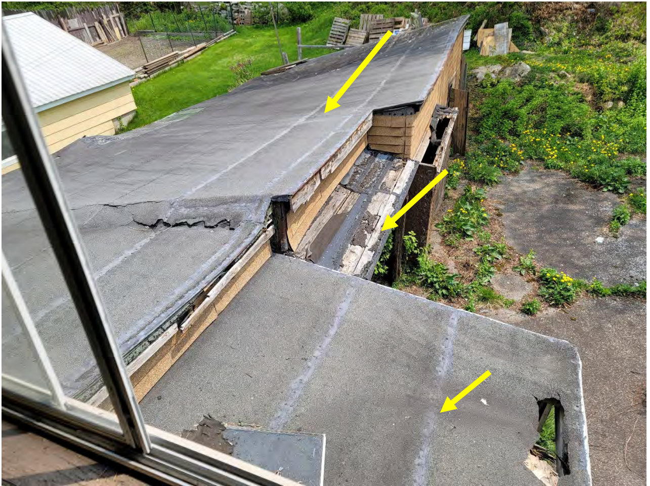
Garage Shed roofs with ACM Mastic/cement.
