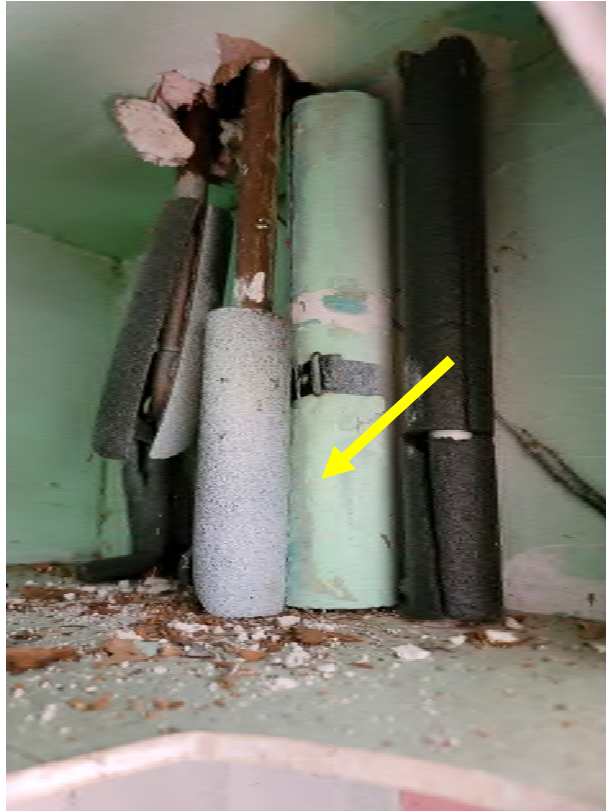
Air cell (ACM) pipe insulation 1 st floor, bedroom 1, closet above shelf.
