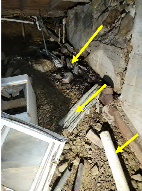
Air cell (ACM) pipe insulation on basement floor.
