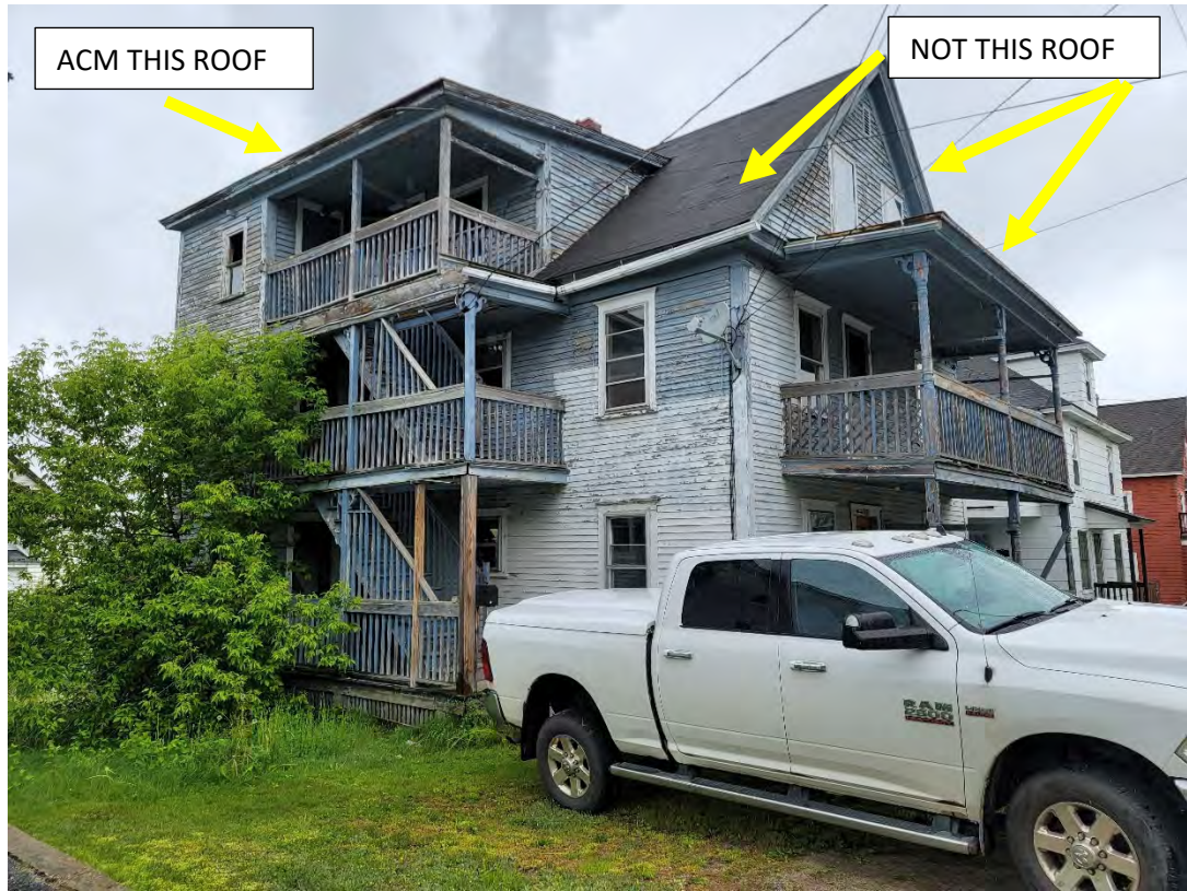
ACM roofing on south porch and "bump out" roof.
