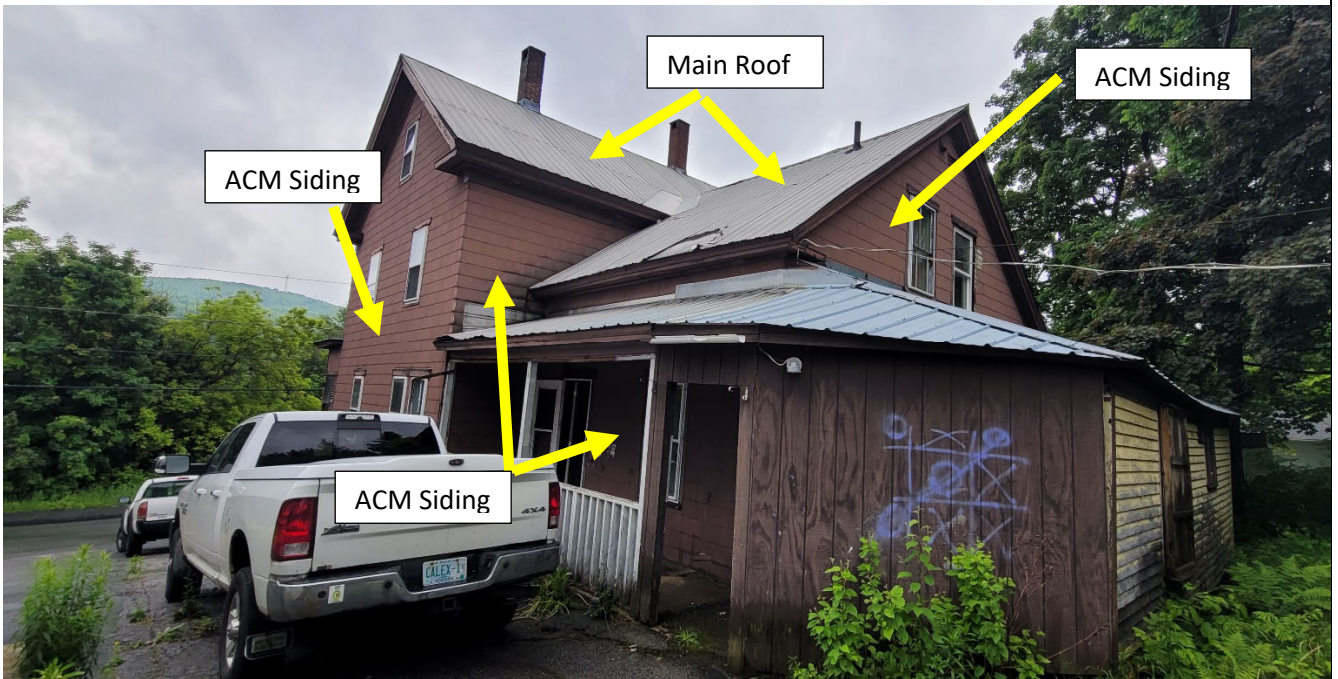
Cementitious (Transite) siding and roof designations.
