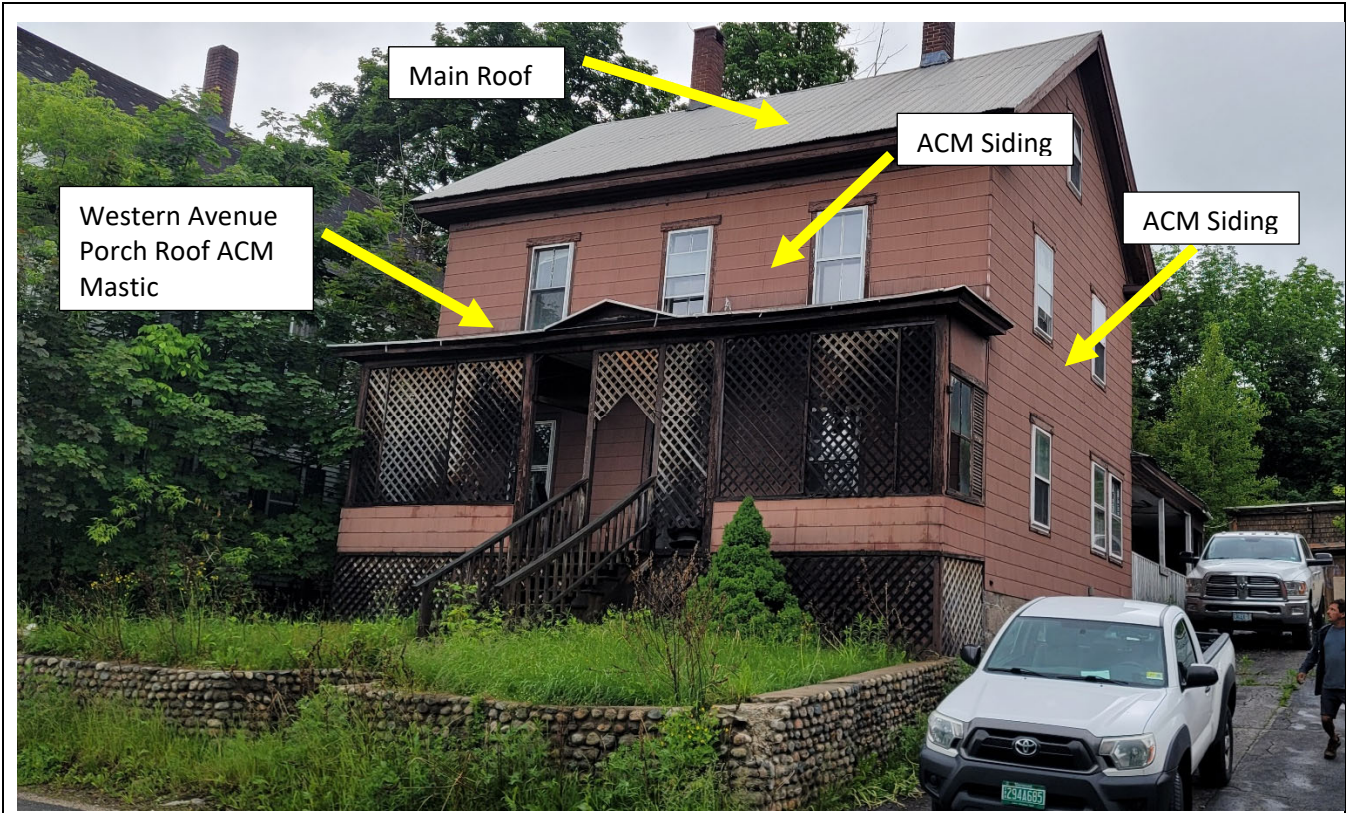
Roof designations and Cementitious (Transite) ACM siding.
