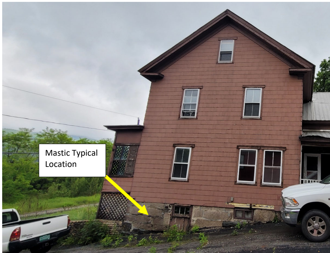
Asphaltic Foundation Mastic (typical).
