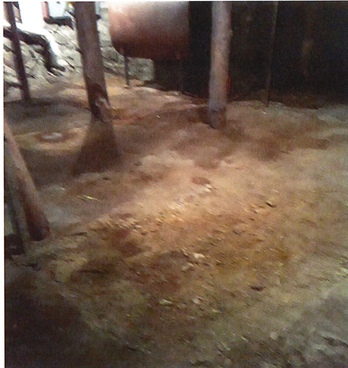
Dirt floor basement where water will pool and filter into ground
