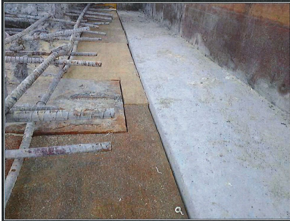
Photo 4: Contractor finishing the concrete at the east abutment.
