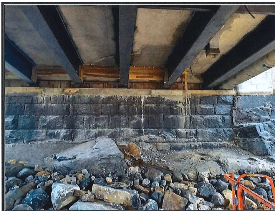
Photo 2: Forms at deck end.
