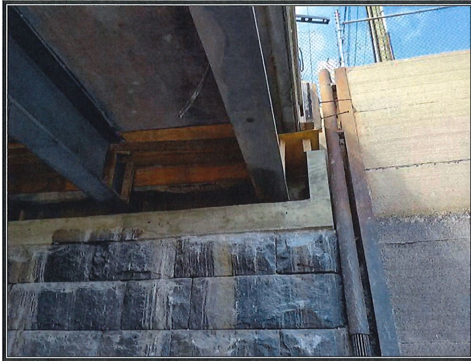
Photo 3: Stone re-set at northeast wingwall.
