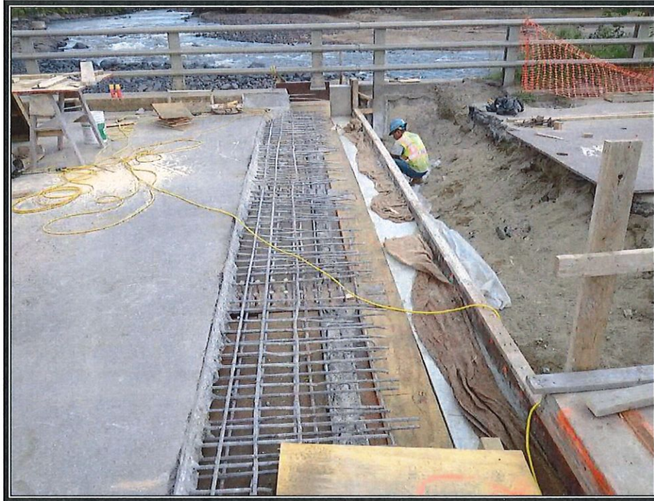
Photo 1: Forms at existing backwall cap.
